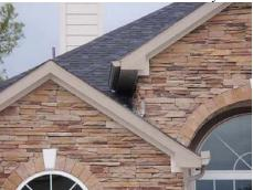
R – At locations where sloped roof shingles meet sided or masonry walls, step flashing should be installed here rather than J type flashing. You should know that siding and shingle companies are moving to void the warranties of their products if "step" flashing is not used:
