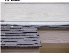
Partial guttering is installed. Full gutters are recommended for all eaves.
