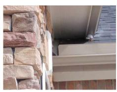
Comment – the flashing at the left side of the entry is very poor workmanship.
