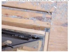
R – the patio door center post has apparently been damaged – the repair is poor with joints not fitting properly – the issue is that these are fully exposed to weather and will deteriorated rapidly – the entire jamb should be replace.
