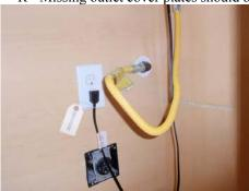
Dryer electric outlet – the screws for this outlet, when provided a ground, will transmit electric current - although not required by code, I recommend that the metal plate and screws be replaced with a plastic plate and screws to reduce the chance of electric shock.
