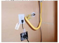
The supply system used in this home is PEX piping with a Manabloc manifold, the ASTM numbers were not accessible. This piping is not new but is relatively new to
